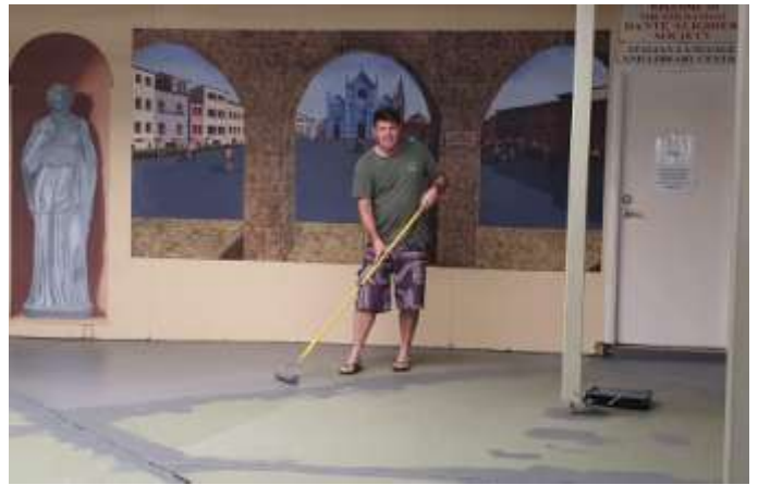
Marco rolling paint on prepared pavement
