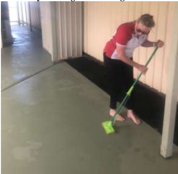
Mopping and drying floor prior to repainting
